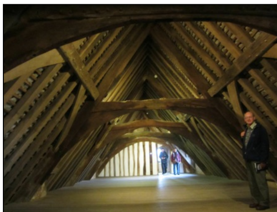
Fig 2. Beamed Attic Roof
