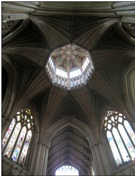
Fig. 5 Looking up into the Octagonal tower and lantern
