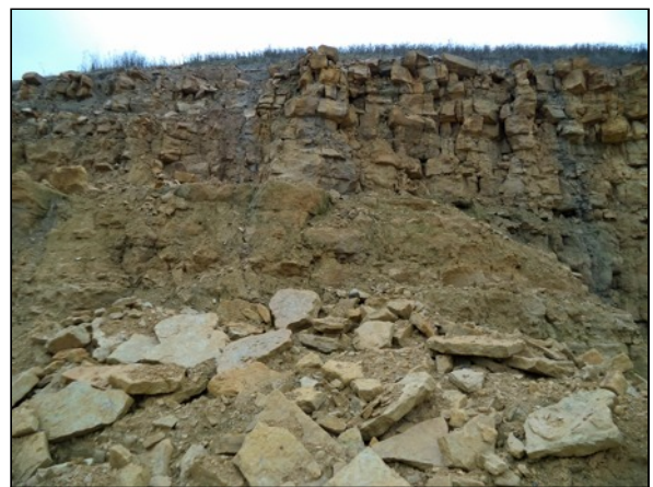
Fig 4 Toppling Failure is likely
